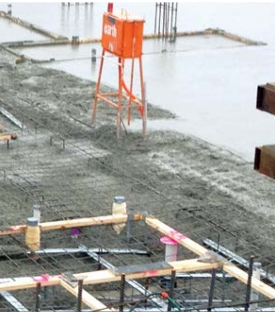
Concrete pour at Sandyhill Apartments
