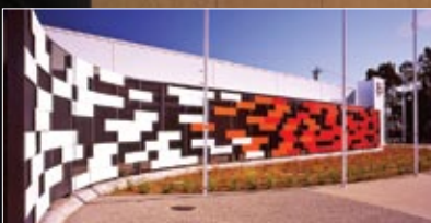
Coffey Projects delivers top class sporting facilities
