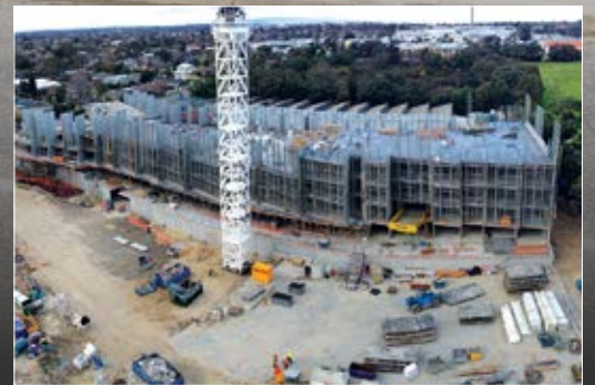
Sandyhill Apartments structure.
